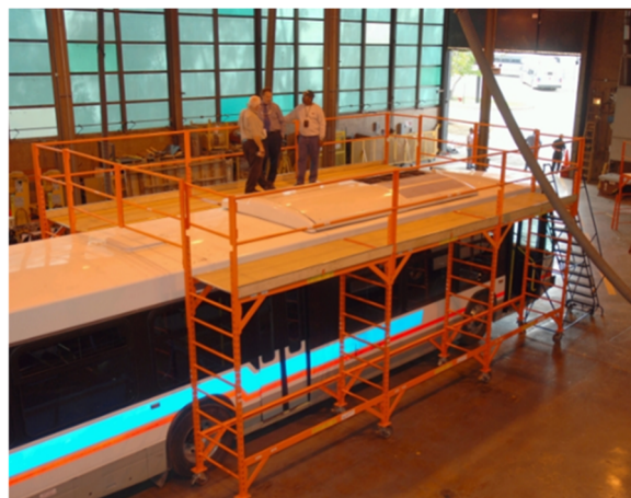
PHOTO-04: BUS SCAFFOLD SYSTEM
