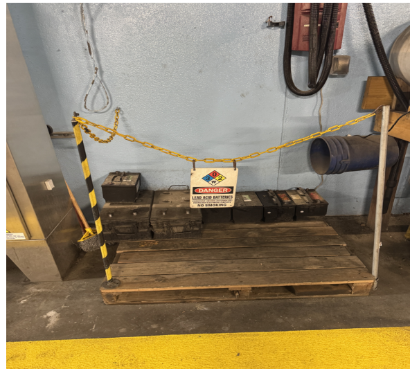
EQUIP-03: BATTERY STORAGE – WITHOUT SPILL CONTAINMENT
