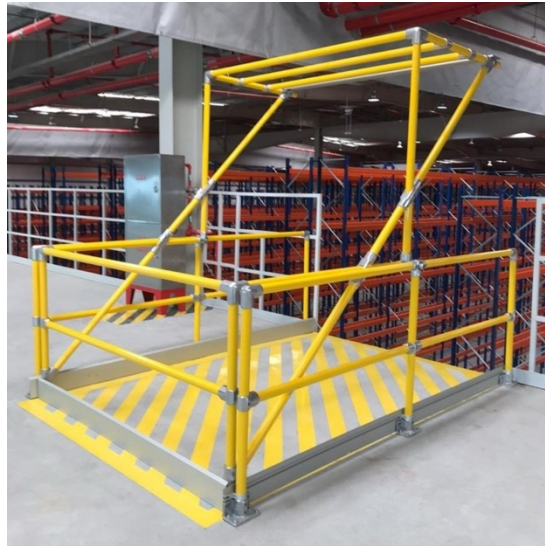
PHOTO-02: EXAMPLE OF GUARDRAIL SYSTEM
