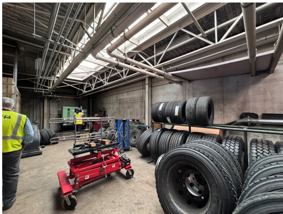
ARCH-10: TIRE STORAGE IN MAINTENANCE MEZZANINE
