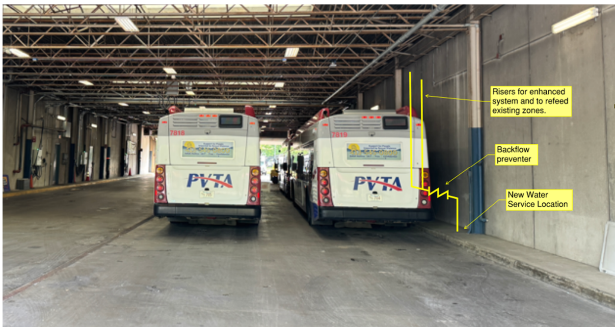
PHOTO-01: POTENTIAL LOCATION FOR NEW FP SERVICE (IT MAY BE THE NEXT COLUMN BAY, BUT THIS REPRESENTS THE INTENT OF OUR THOUGHT)
