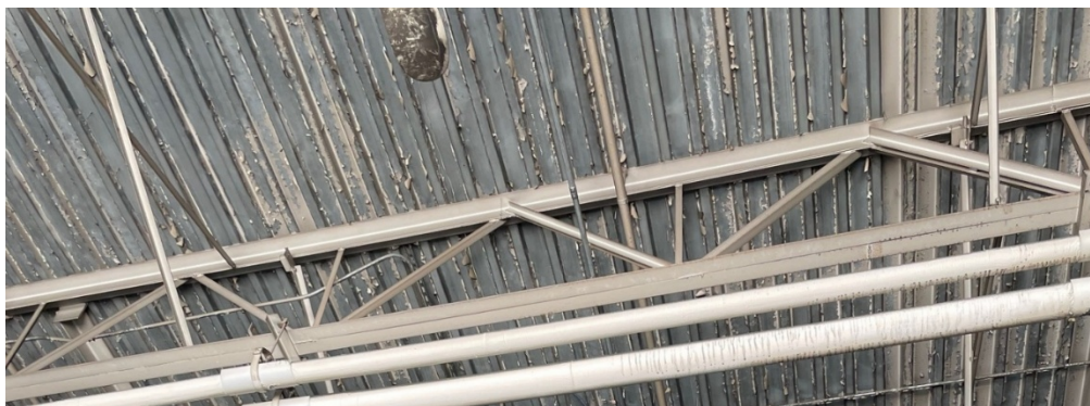
ARCH-03: EXISTING METAL DECK
