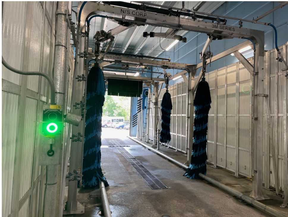
ARCH-07: EXISTING BUS WASH
