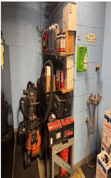
EQUIP-03: BATTERY STORAGE – WITHOUT SPILL CONTAINMENT
